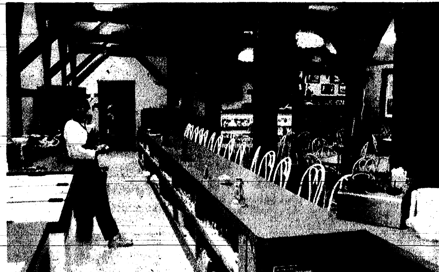
THE OLD POST AND BEAM CONSTRUCTION of the former Cole's Elevator in Gregory can be seen in the new Scoops Ice Cream and Deli. The kind of pine used in the construction no longer exists in Michigan, says renovator Duane Innes. The ice cream shop has a friendly decor and atmosphere.
